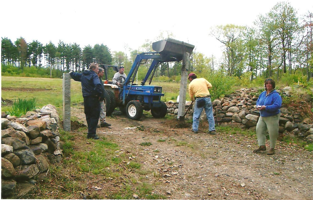
Jon Sanborn & Mark Latham Install The Granite Entrance Posts
