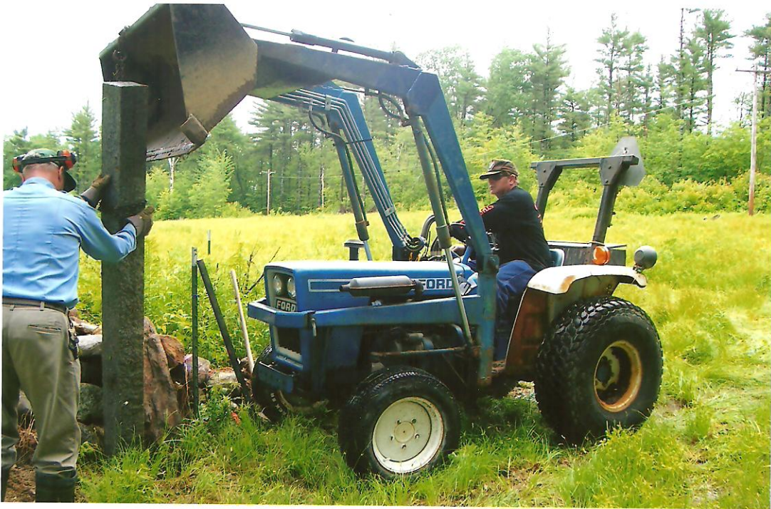
Peter Hibberd & Jon Sanborn Install The Exit Granite Posts
