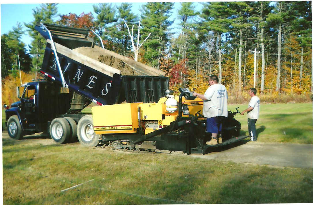
Laying The Top 6 inches of Hard-Top
