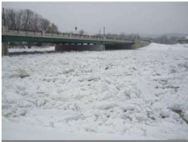
March 2011 Ice Jam at NH Route 175A bridge across the Pemigewasset River
