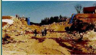
Alton dam breach, 1996
